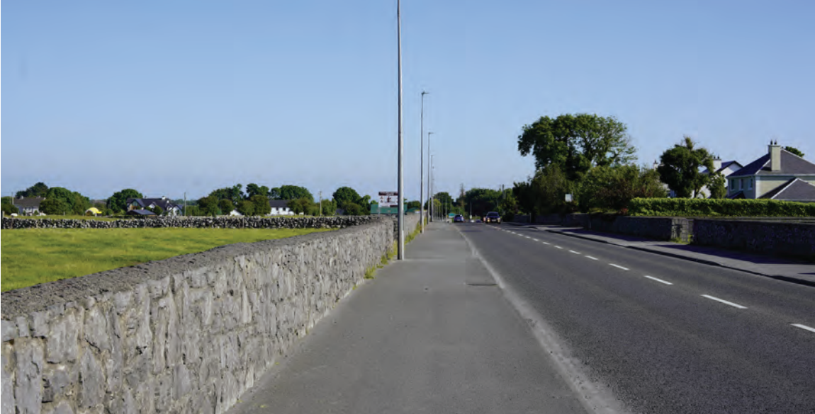
Parkmore Rd looking south
